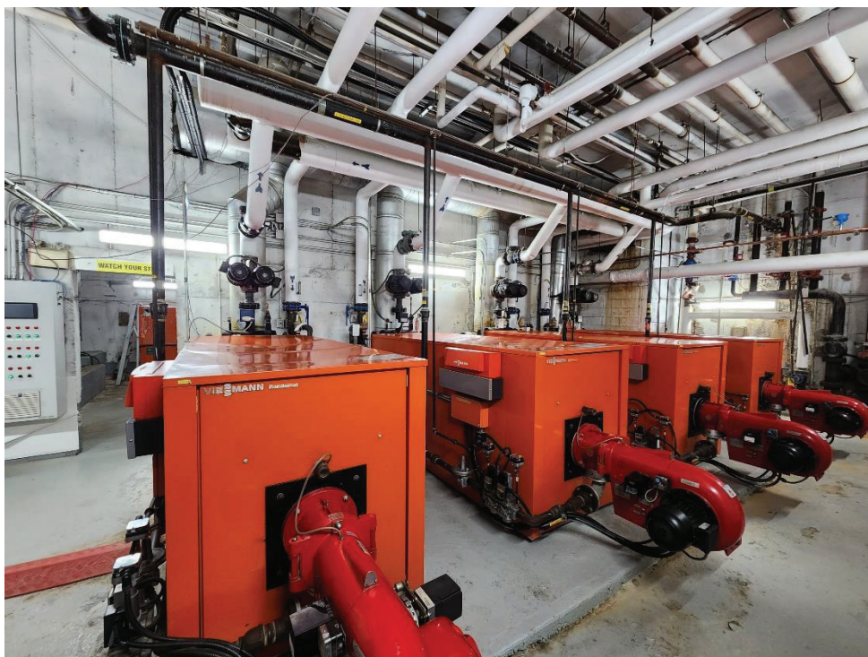
Photograph 7: View of natural gas-fired boilers in basement boiler room
