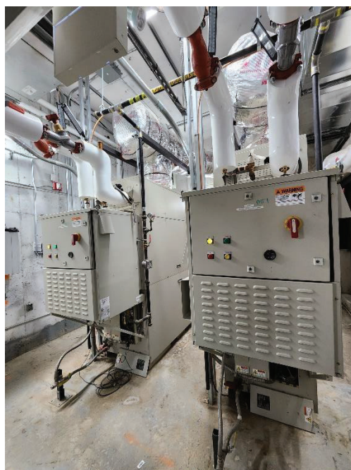
Photograph 10: Natural gas-fired generators in the basement generator room
